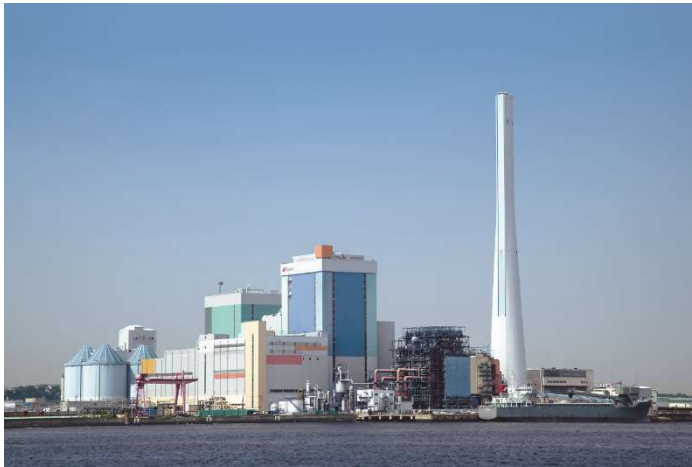
Figure 8: Photo of Isogo Power Station
