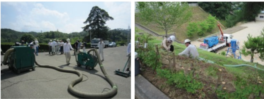
Fig. 3. (Left) Sandblast method ( 8 \mu\text{Sv h}^{-1} \Rightarrow < 0.7 \mu\text{Sv h}^{-1} ). (Right) Electric cutter method ( 3.5 \mu\text{Sv h}^{-1} \Rightarrow 1 \mu\text{Sv h}^{-1} )
