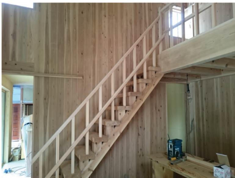
Fig. 3. The heartwood is placed side by side to form a wall.
